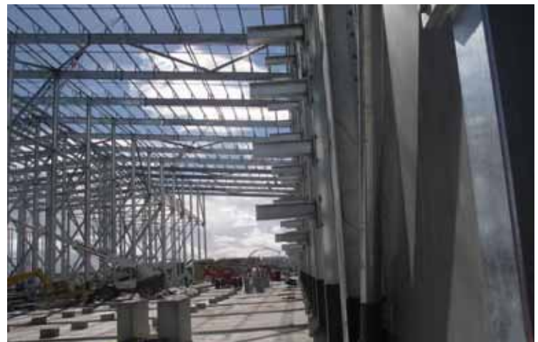
Structural steel showing extra corrosion protection at base of columns
