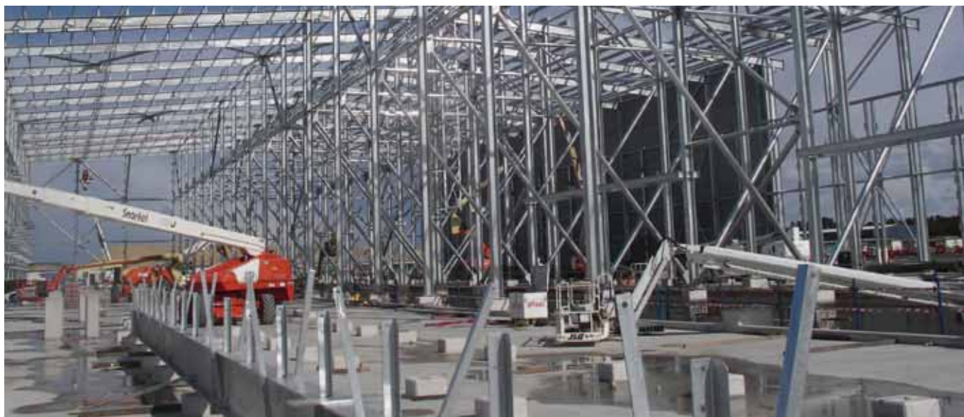
Structural steel at the Sydney Desalination Plant
