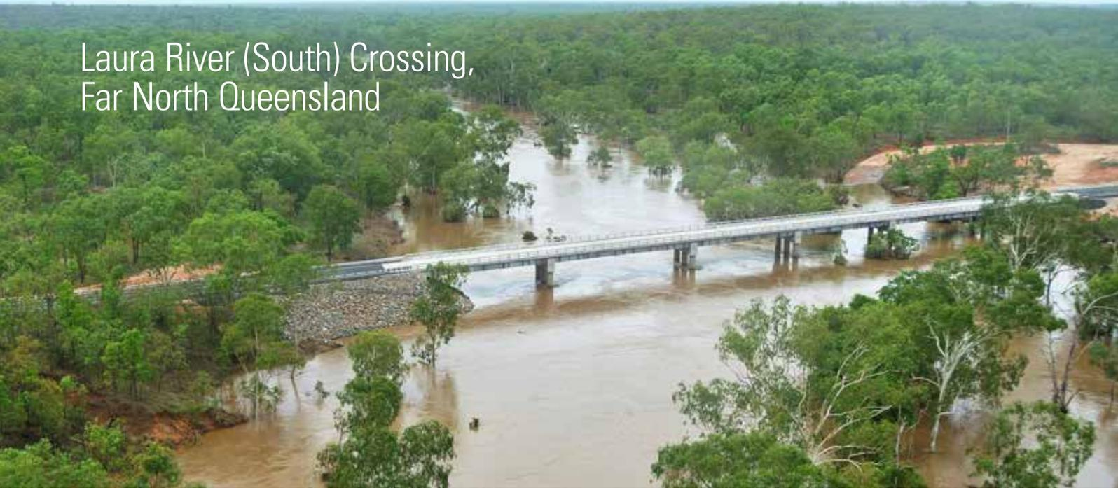
The ability to supply lighter weight components for a remote location and construct a continuous superstructure to achieve structural efficiency, also lending itself to slimmer design less affected by water flows during extreme floods, prompted the new bridge over the Laura River to be built predominantly in steel.
