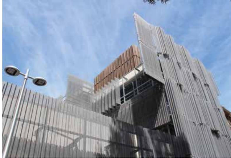
The HDG steel will easily achieve the 25 year design life for the building façade with minimal maintenance.
