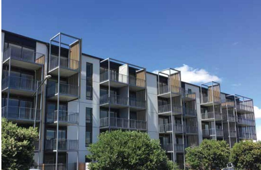
The use of a duplex system built on the resilience of hot dip galvanizing has enabled the use of architecturally exposed structural steelwork (AESS) in a relatively corrosive river land environment.
