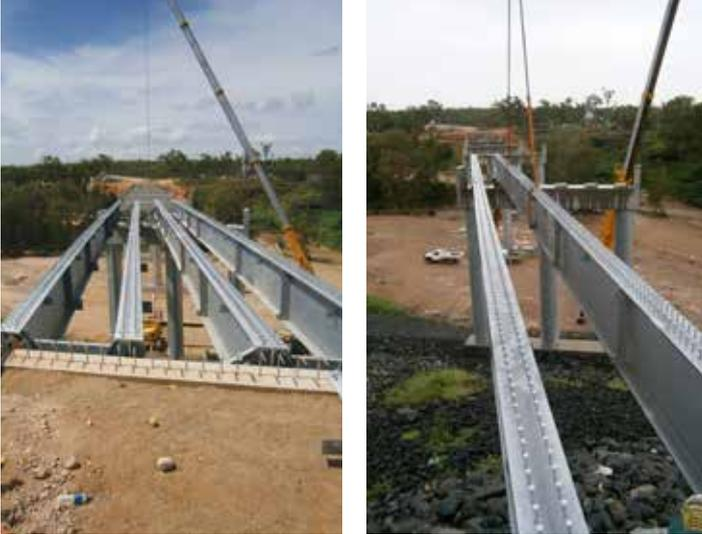
Over 6000 bolts with some beams pre-spliced before erection and some mid span splices were conducted in situ
