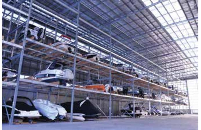
The hot dip galvanizing of the support structure and racking system of an innovative dry storage facility for watercraft located on a flood prone site at Sydney's Rozelle Bay will optimise the operational life of the facility and also help to reduce water traffic and pollution.
