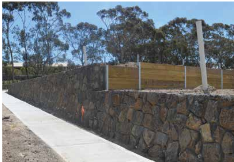
Part of the 750m long retaining wall
