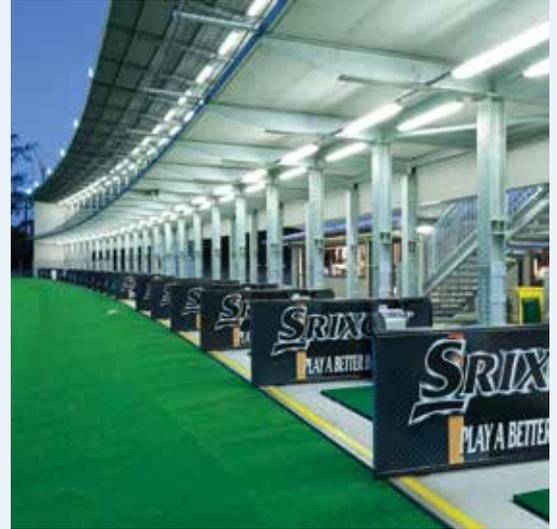
Hot dip galvanizing (HDG) applied to the entire structure of a driving range practice facility of a new golf centre in Sydney's northwest transformed what was a disused and derelict industrial brick pit and waste site into a modern and enduring sporting venue.
