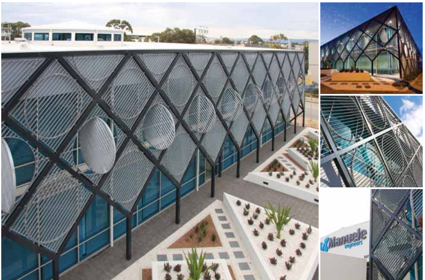
Manuele Engineers Steel Facade Building, North Plympton South Australia
