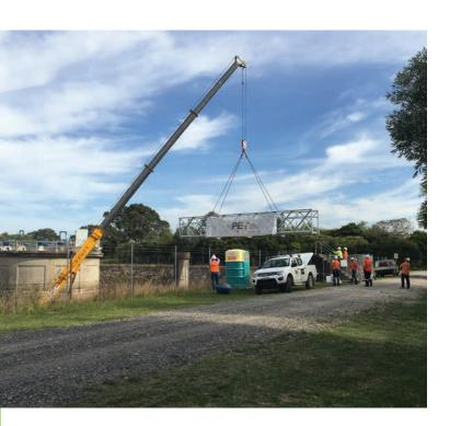
The new bridge consists of two 12.3m long, 1.5m wide fully welded truss frames that were each galvanized in a single dip.
